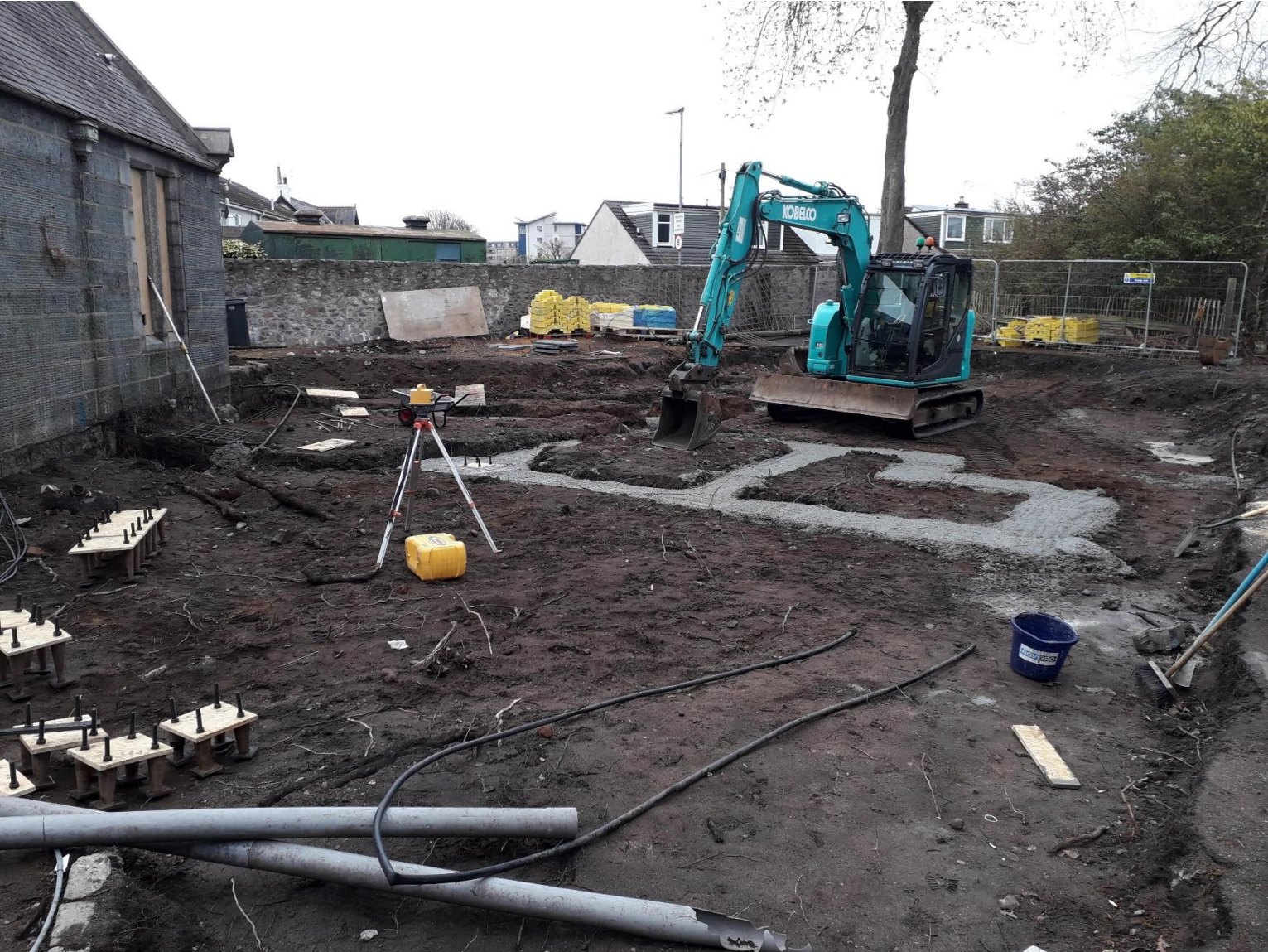
Duthie Park – Progress Picture
