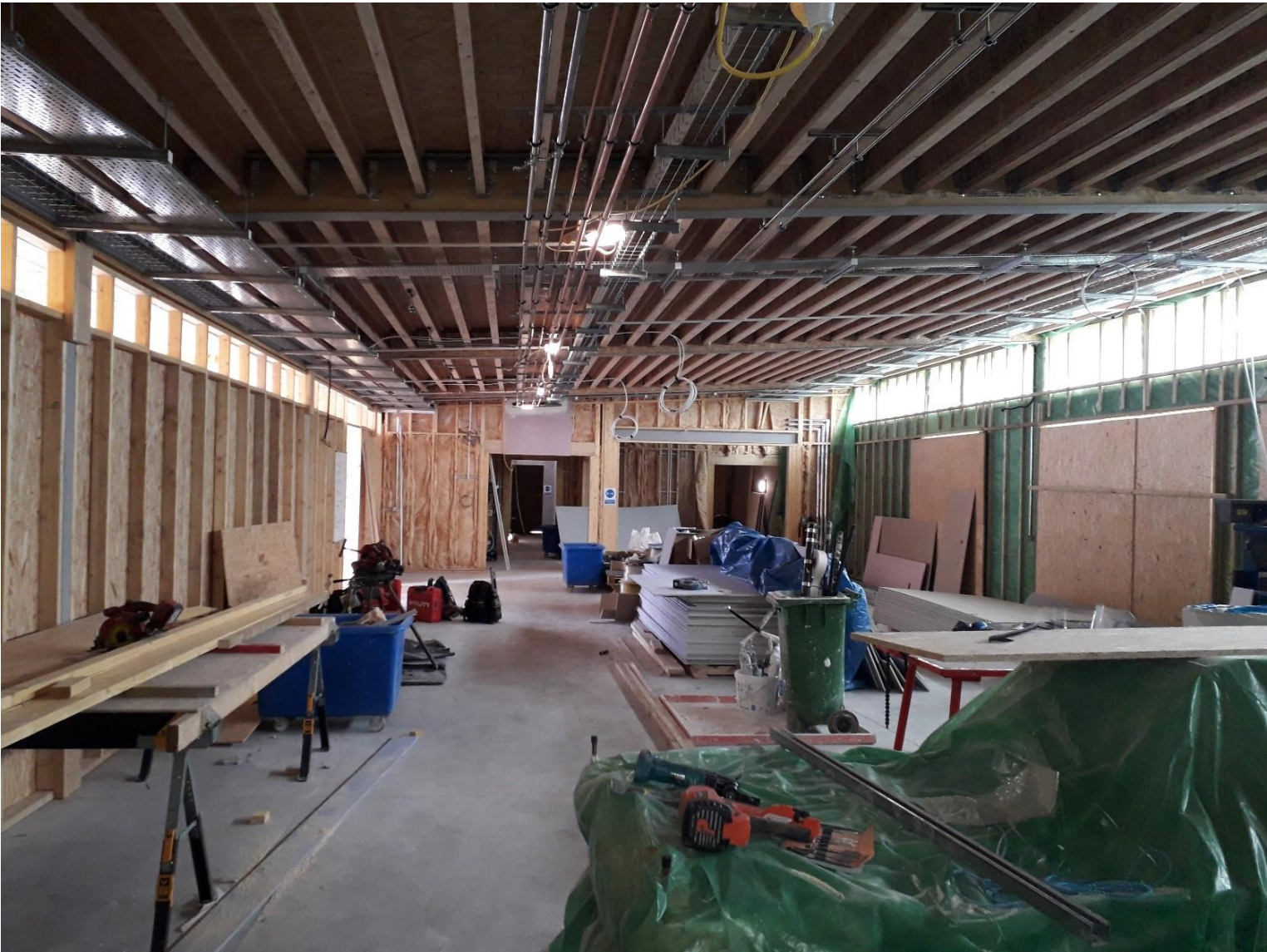
Broomhill – Progress Picture
