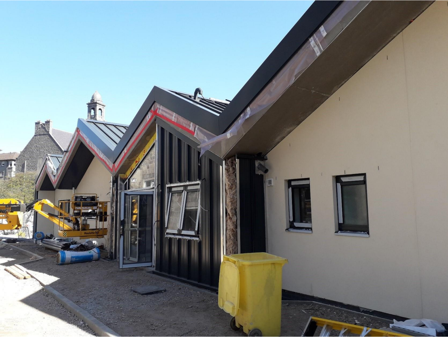
Gilcomstoun – Nearing Completion
