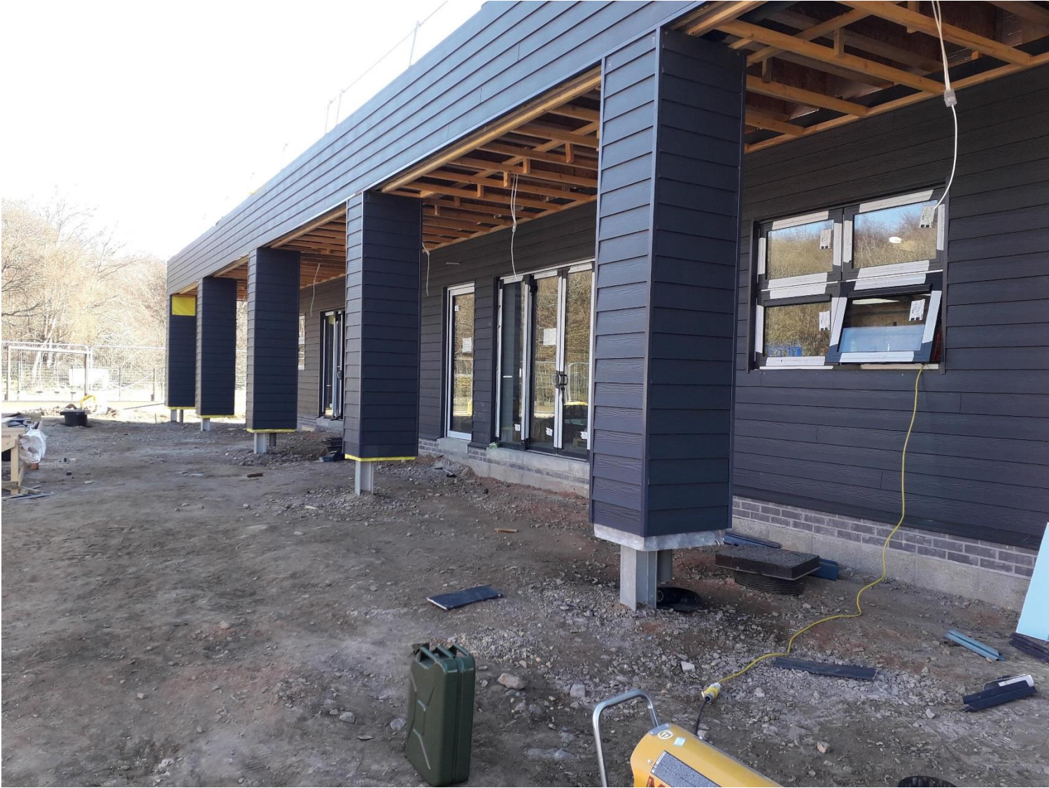
Cults – Nearing Completion
