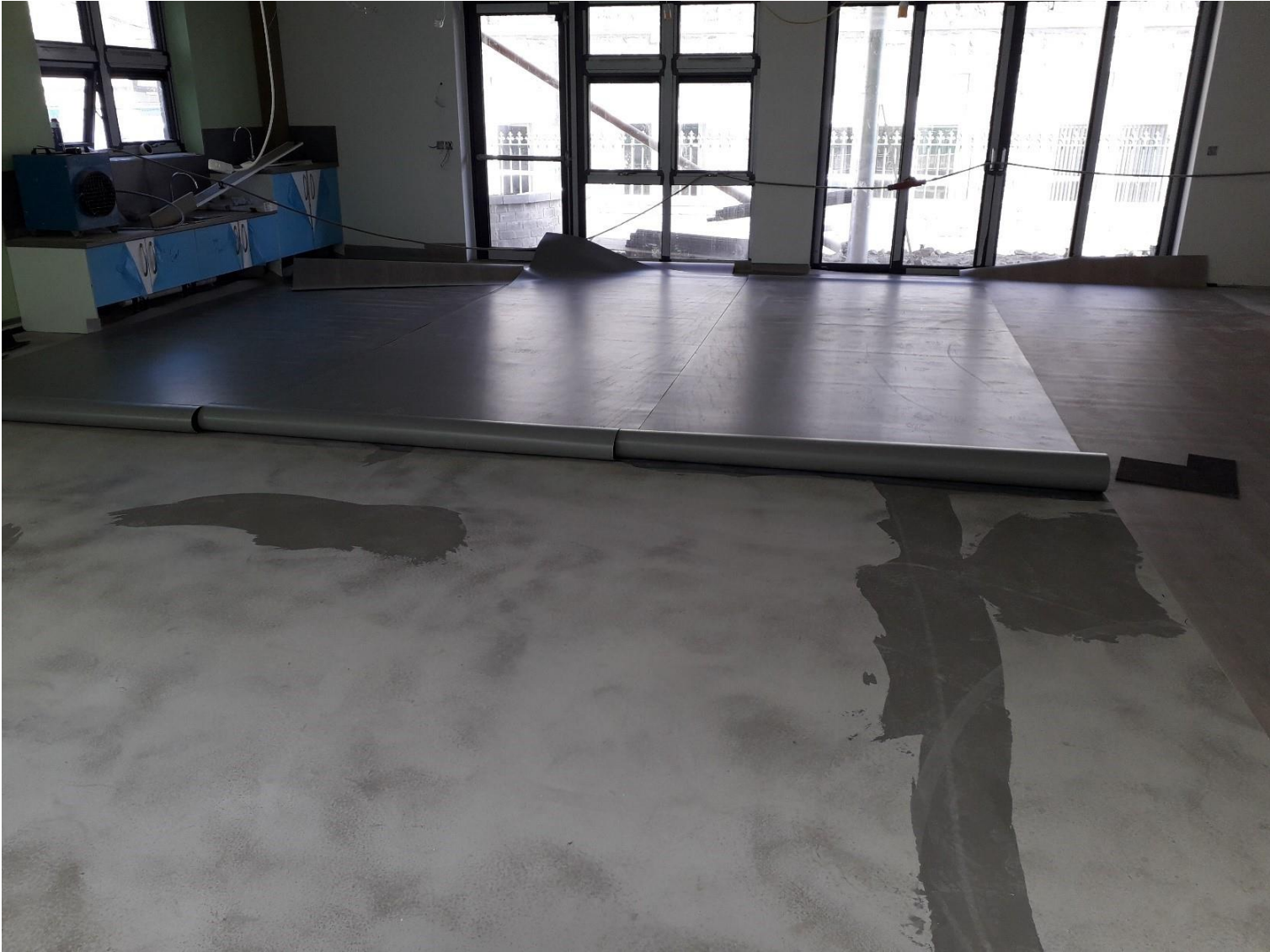
Woodside – Nearing Completion
