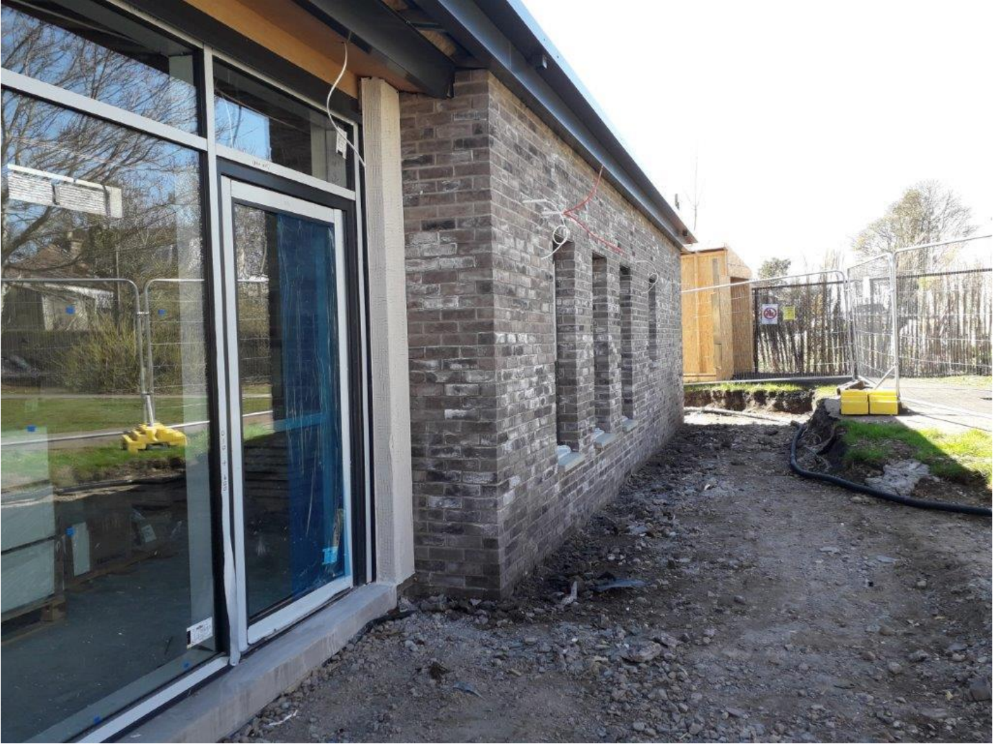
Culter – Nearing Completion
