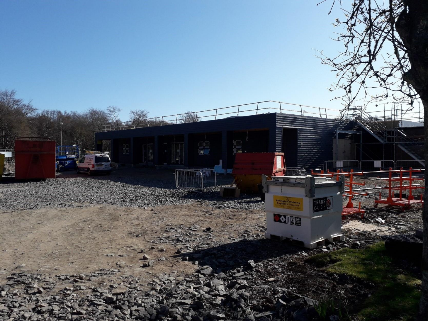
Cults Nearing Completion
