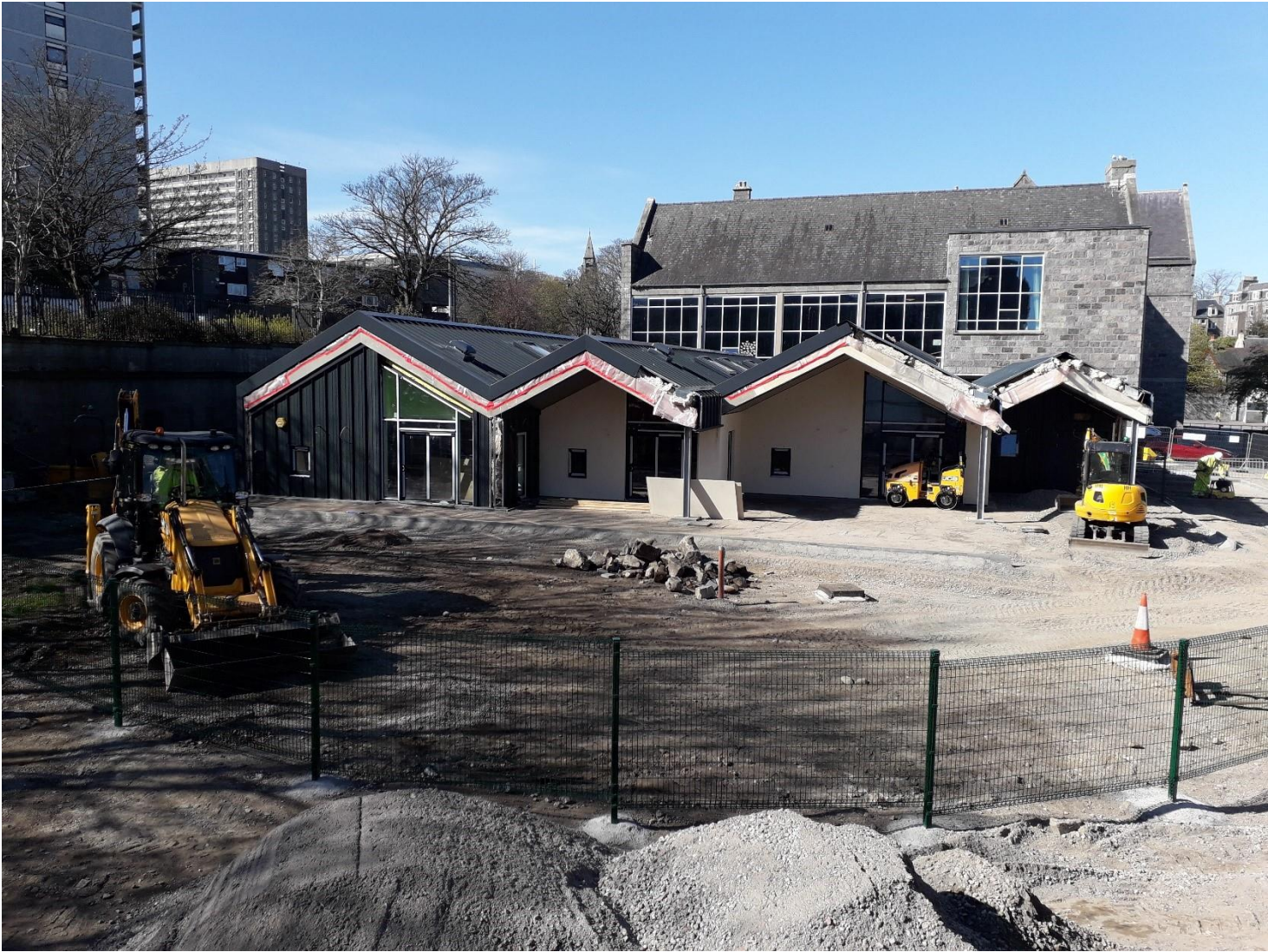
Gilcomstoun – Nearing Completion
